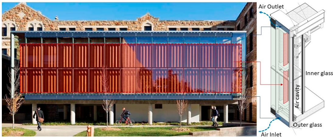
Figure 2. Double skin façade building at the University of Kansas (source: https://studio804.com/ ).
