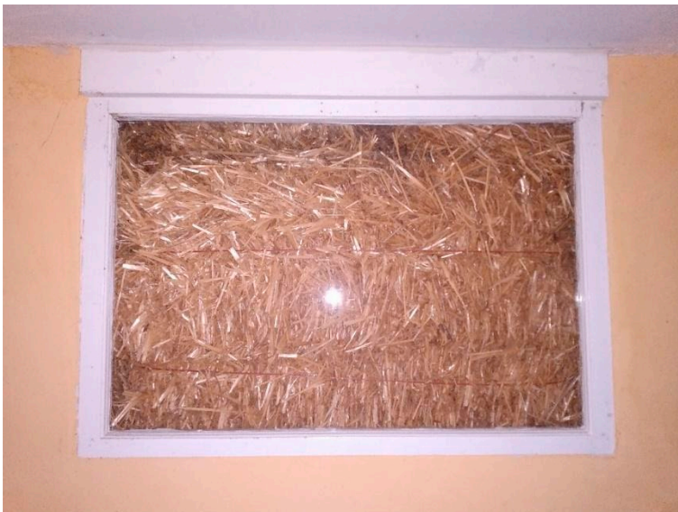
Figure 2. Truth window, interior wall of straw bale structure. Source: Photo by author, author’s garage/studio, Ogden, UT.
