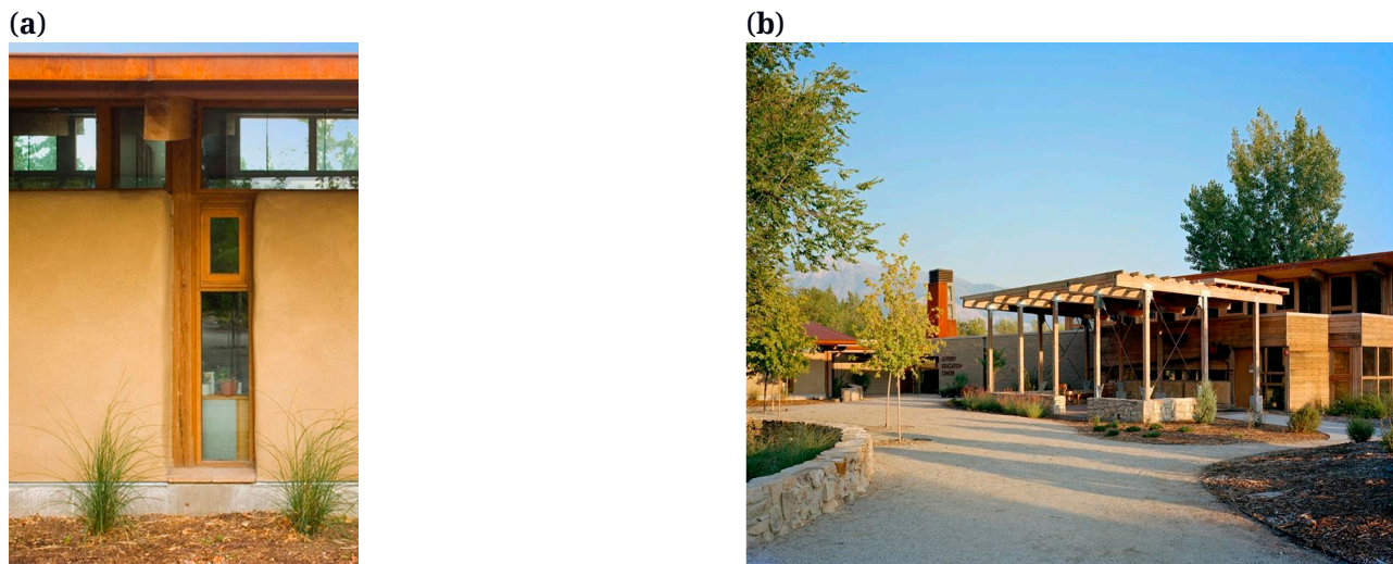
Figure 3. (a) Ogden Nature Center Education Building. Source: EDA Architecture [74]. Close-up view of straw bale wall at left side of entry. (b) Ogden Nature Center Education Building. Source: EDA Architecture [74]. Education Center entrance with solar chimney visible at back, left.
