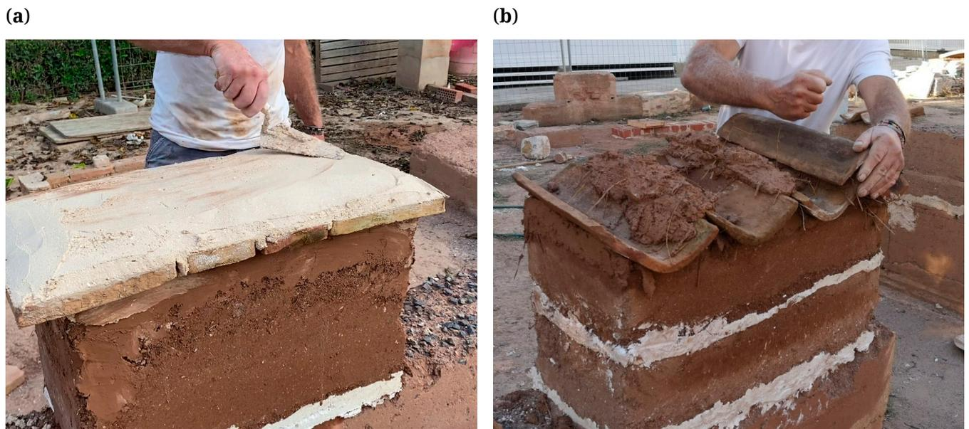
**Figure 5.** Execution process of protective elements on top of rammed earth walls. **(a)** Protective element with bricks and lime mortar on wall T1. **(b)** Protective element with curved tiles and earth mortar.
