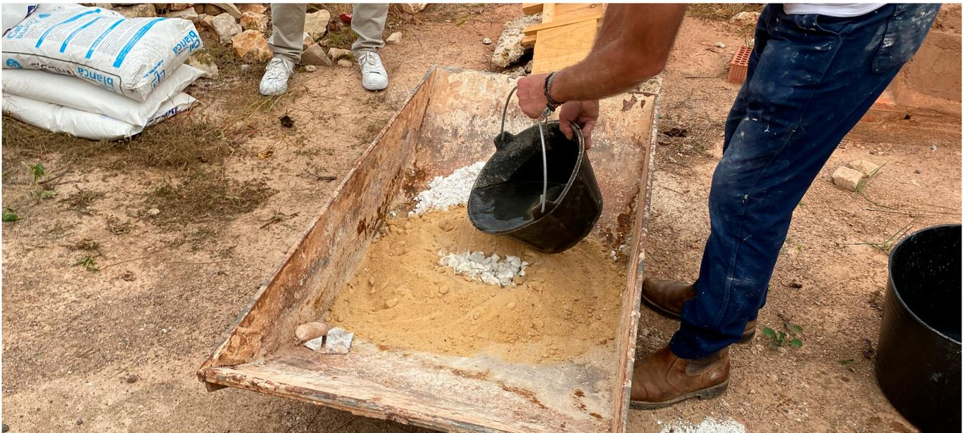
**Figure 1.** Quicklime slaking process using the traditional method to prepare a mortar, part of the construction experiments carried out in this study.
