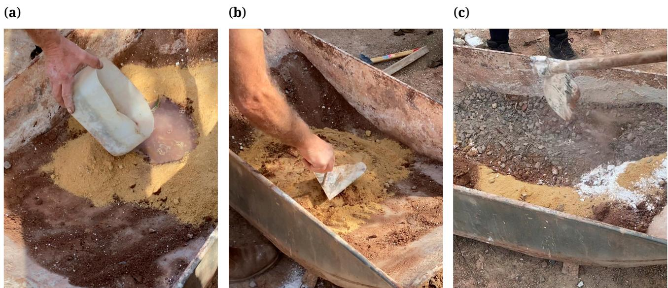
**Figure 6.** Execution process of the used mix. (a) Mixing quicklime with water to begin the process. (b) Process for slaking lime during the time needed for the correct hydration to take place. (c) Adding the rest of the mix and water to ensure a suitable consistency.
