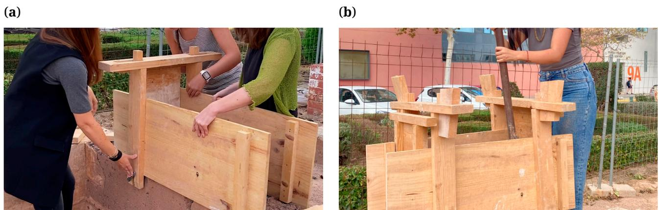
**Figure 4.** Execution process of rammed earth walls. (a) Assembly of formwork on pre-existing walls built on brick plinths. (b) Execution and tamping of rammed earth walls.
